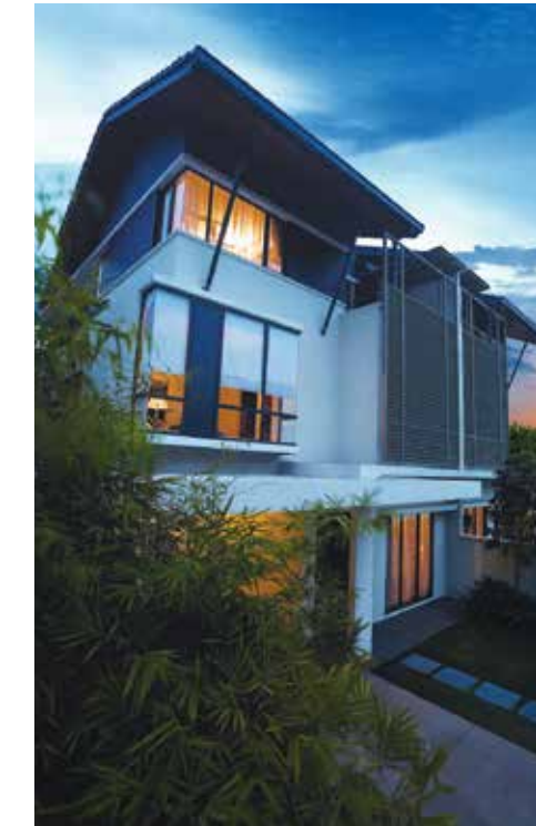
Idamansara Damansara Heights
